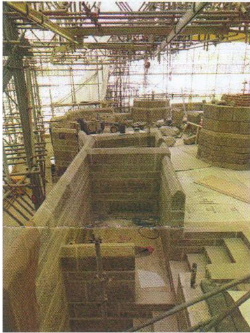
Parapets rebuilt on the central tower
